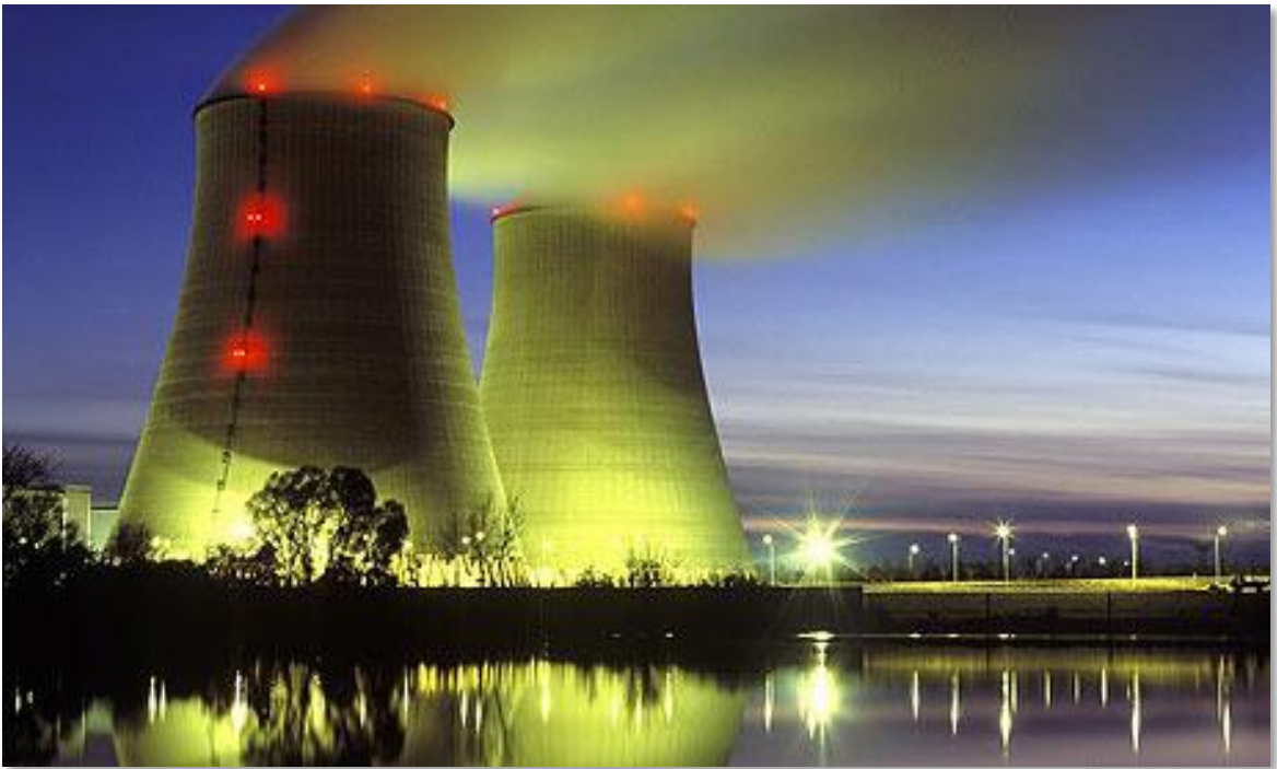
The nuclear power plant in Belleville sur Loire, France. Photograph: Herve Lenain/Corbis
