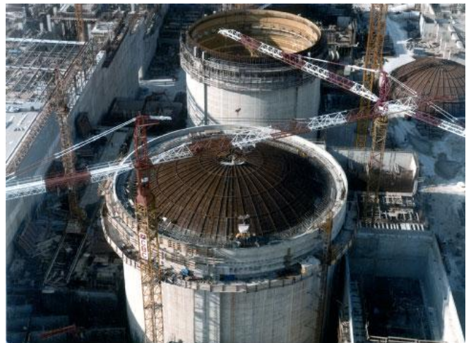
Tricastin Power plant – efreyssinet- Association
